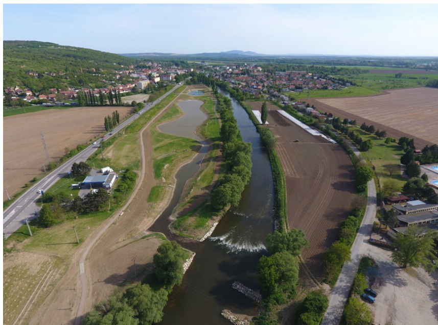
Figure 5 Židlochovice: Aerial view of the newly established floodplain park along the Svatka River Source: Archive of the municipality Židlochovice
