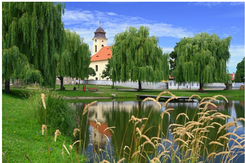
Figure 2 Kostelní Lhota: The Church of the Assumption of the Virgin Mary, a significant cultural monument of the village, which has been sensitively restored in recent years Source: Archive of the municipality Kostelní Lhota
