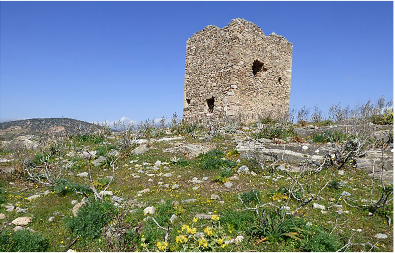
Figure 2 The Dagla's Tower at the top of the hill Source: Authors archive
